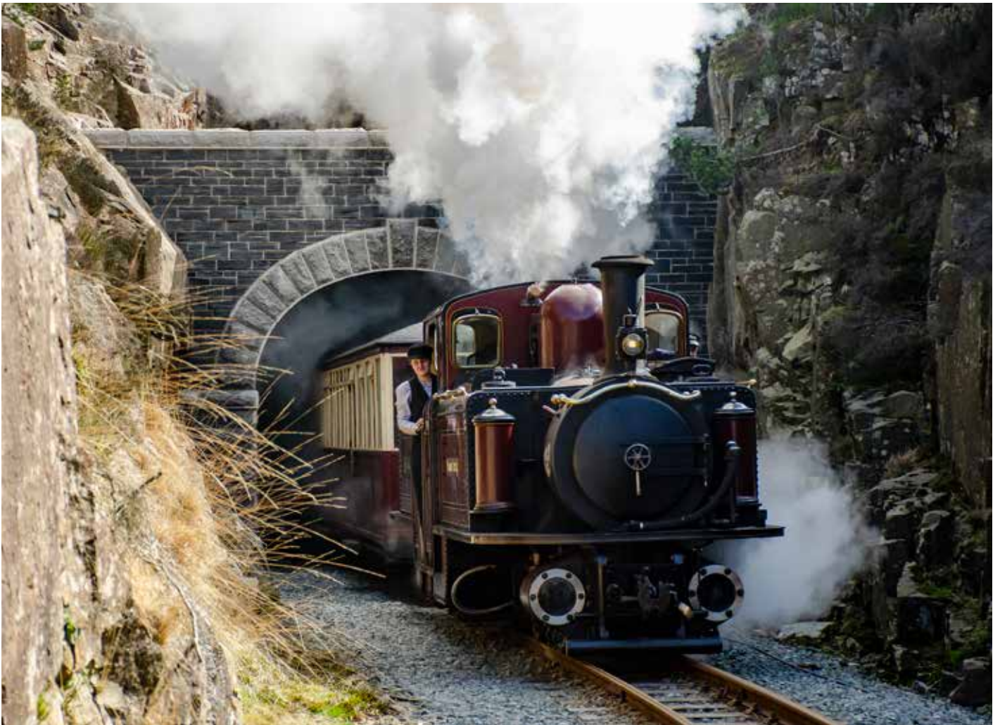
Moelwyn Tunnel North Portal
