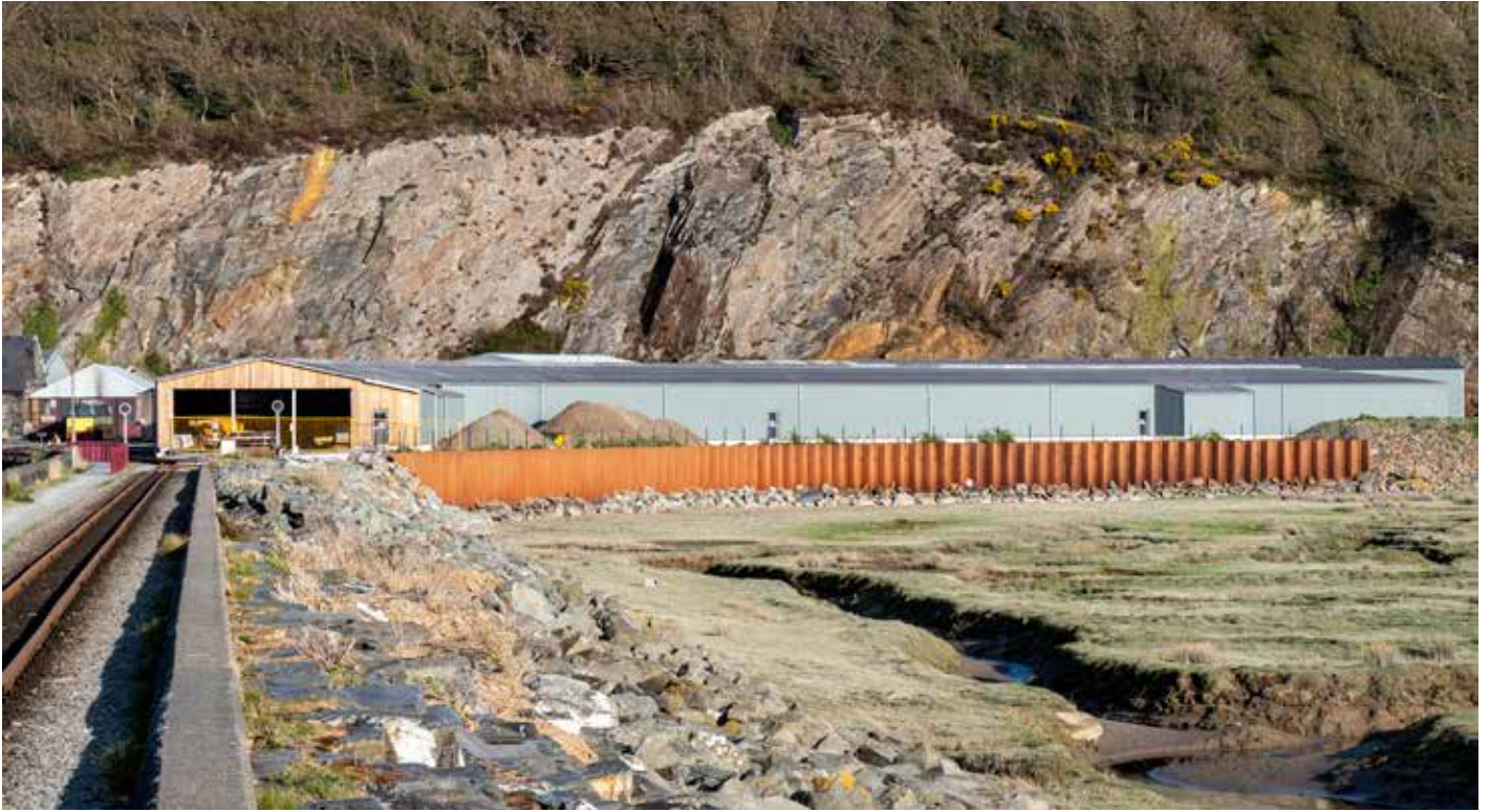
New Boston Lodge Carriage Shed taking shape
